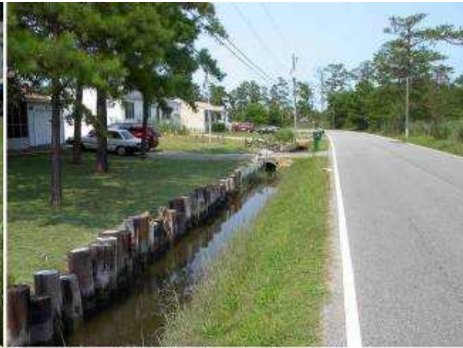
Photos 11–12. Tidal Ditches in Poquoson. Photo 11 shows wetland vegetation in a tidal ditch. Photo 12 shows a wooden bulkhead along the shore of a tidal ditch, to prevent a front yard from eroding into the ditch and blocking drainage (October 2002).
