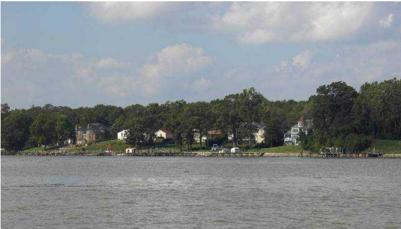
Photo 8-50. Shoreline Armoring along the Potomac River South of Mount Vernon (October 2003).
