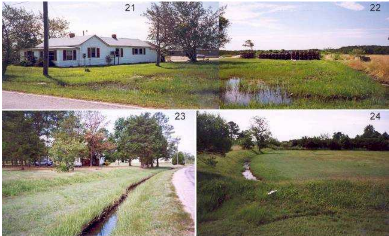
Photos 21–24. Guinea Neck. Photos 21 and 22 are near the end of Maryus Road in Guinea Neck, looking north. The front yard of the home in the foreground is only one foot above the level of spring high water. Two piles of fill dirt can be seen along the home in the background, along with crab pots neatly stacked. Photos 23 and 24 show low dikes, which protect the land behind them during minor storm tides and extreme astronomic high tides. They also show the tidal ditches along the street, with various forms of marsh vegetation. In Photos 21 and 24, people mow the high marsh grasses as if they were ordinary lawns (July 1998).
