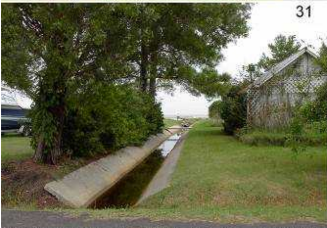
Photos 29–32. Lewisetta, Virginia. Photos 29 and 30 show tidal ditches along the streets of Lewisetta. The concrete-lined ditch in the foreground of Photo 31 conveys water from a ditch along the street to the Potomac River. In the background is a seawall along the Potomac, and a tide gate, which allows the ditch to drain except during high tides. Photo 32 shows low, but somewhat higher, development behind bulkheads along the protected shore on the east side of the community. October 12, 2002.
