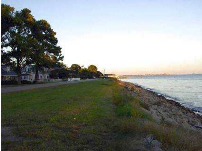
Photo 8-18. South Shore of Hampton. The public has access along this shore, which is protected with a stone revetment.
