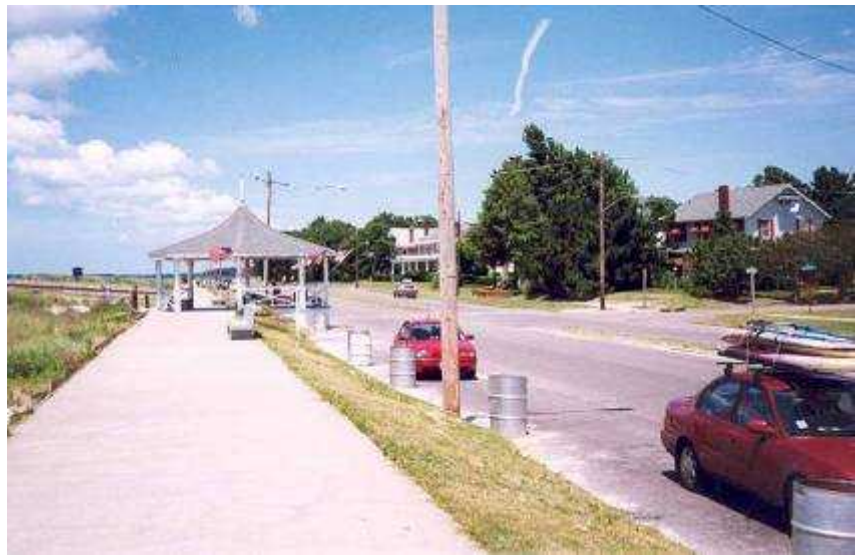
Photo 8-10. Cape Charles, Virginia. Dunes along the beach at Cape Charles are just to the left of the photo, with the primary road along the shore to the right.
