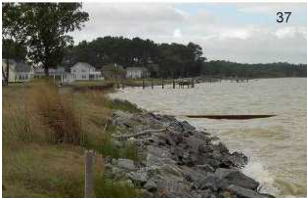
Photos 37–38. Armoring That Protects Undeveloped Land. Photo 37 shows a rock revetment protecting an undeveloped lot in a waterfront community at Newman Neck. Photo 38 shows a revetment protecting undeveloped lands near the VA-3 bridge into Lancaster County (October 12, 2002).
